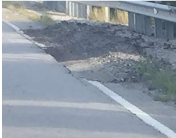
Shoulder failure
