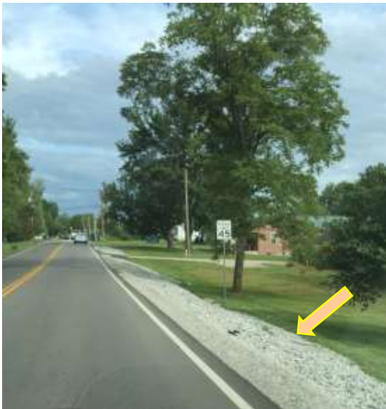
Shoulder widening in Alton area
